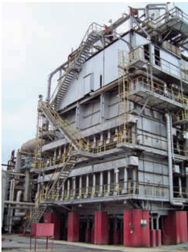
FIG. 1 Pre-revamp view of the primary reformer.
