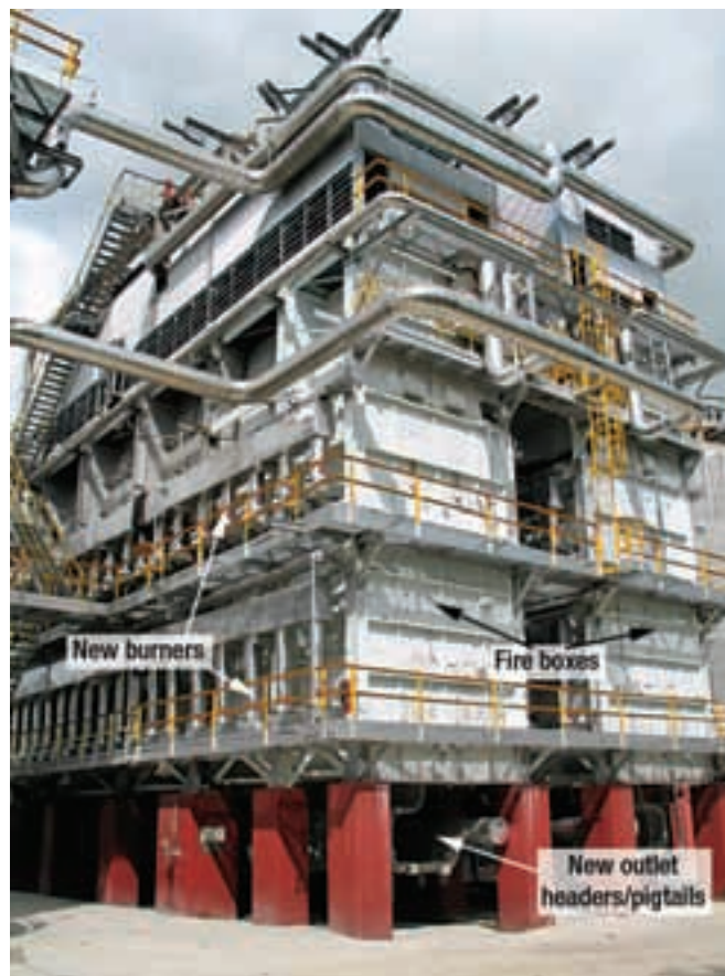
FIG. 8 Post-revamp view of the primary reformer.
