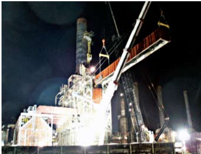
FIG. 7 Lifting of Module 5 during the revamp of the reformer heater.
