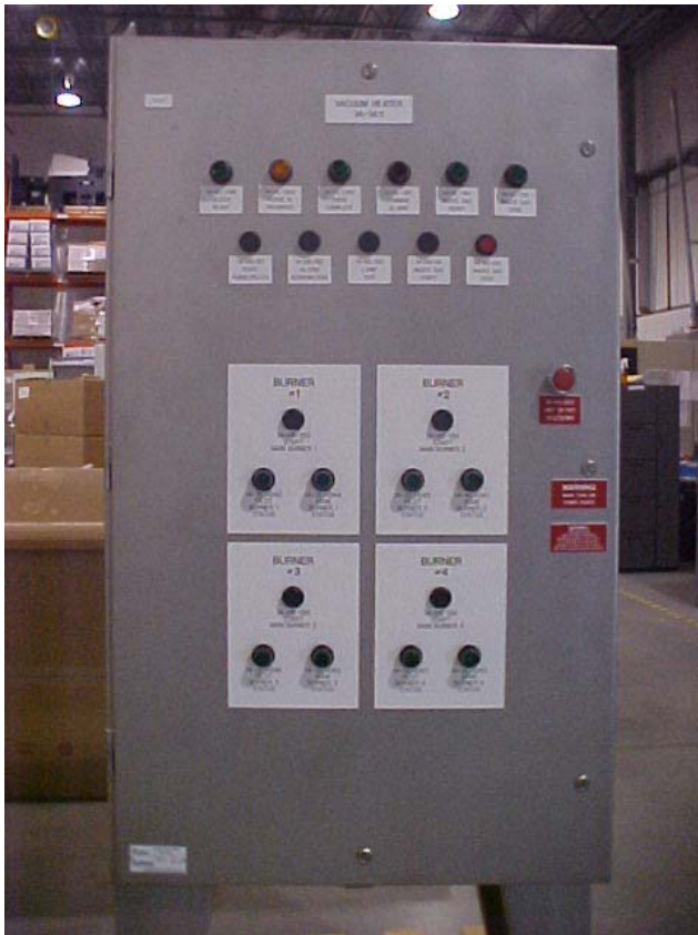
PLC Panel with Lights and Push Buttons
